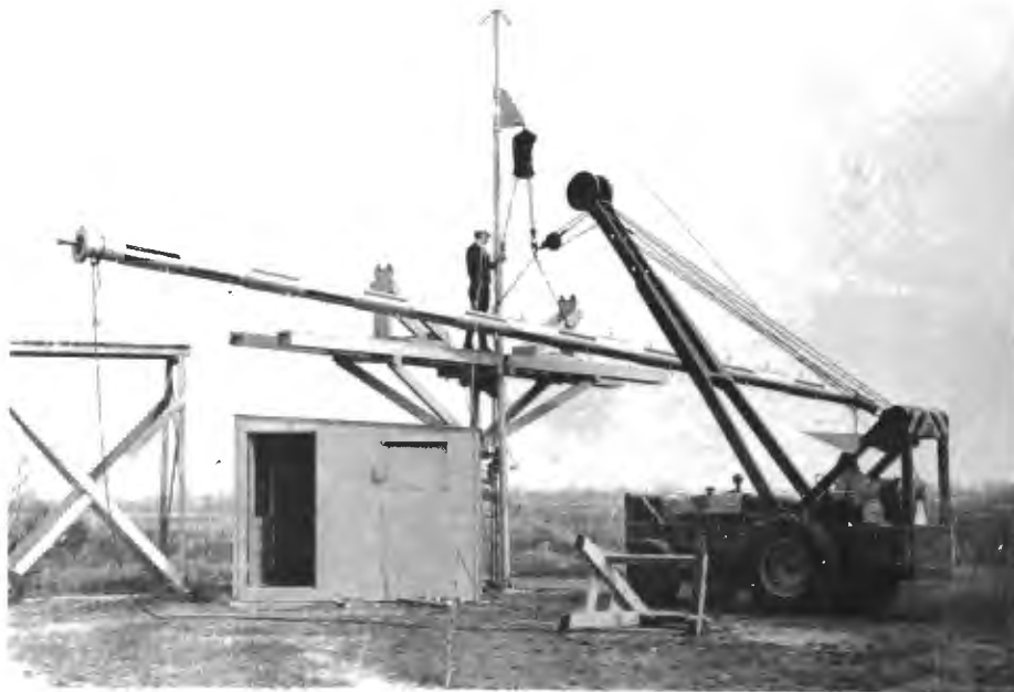
FIG. 11. Crane in operation.
