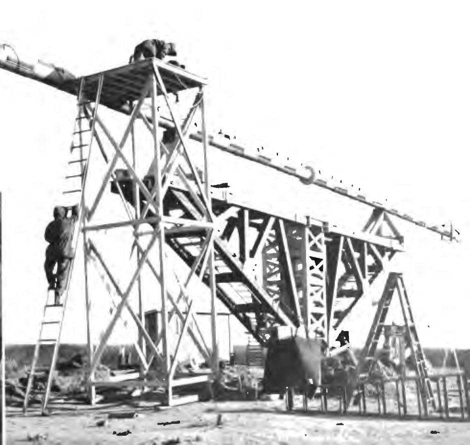
RCA engineers inspect the flanged joint at which the two sections of the ultragrain antenna have been assembled prior to hoisting the antenna on top of the turntable for pattern and gain measurements.
