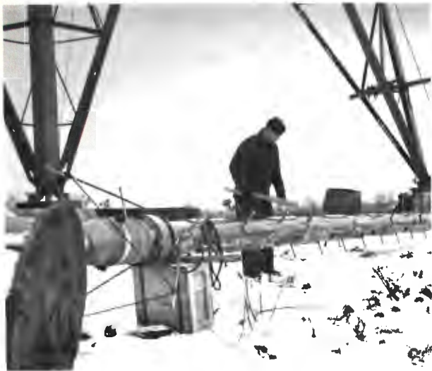
Top antenna section at the tower base. The weather has cleared, but the cold continues.
