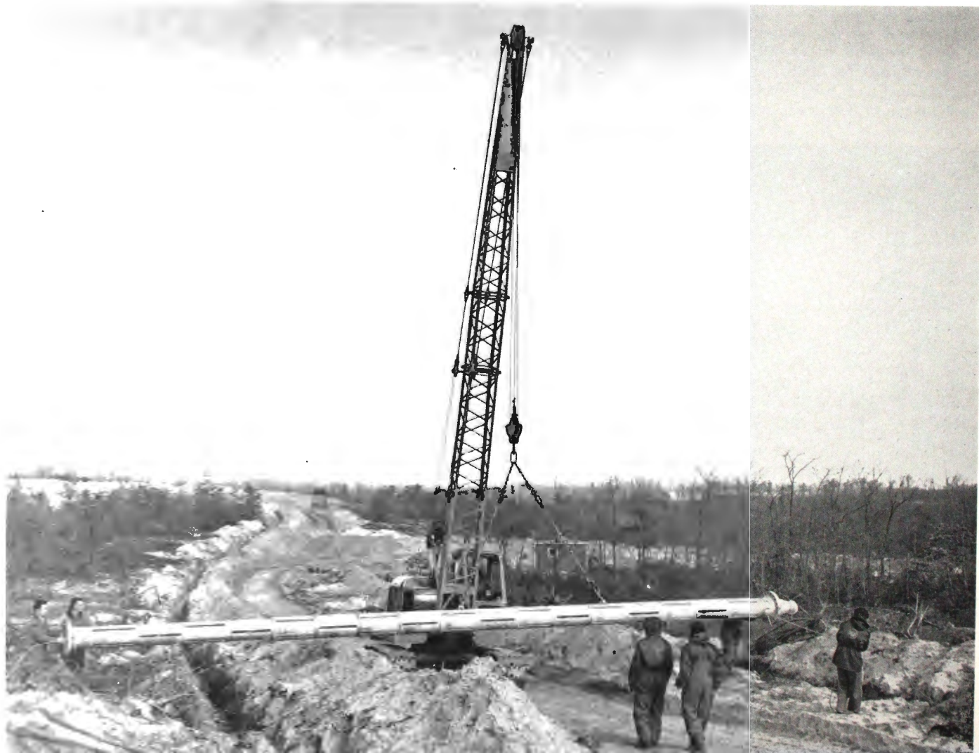
One section of the fabricated antenna is moved up a newly bulldozed road to the Gibbsboro site.
