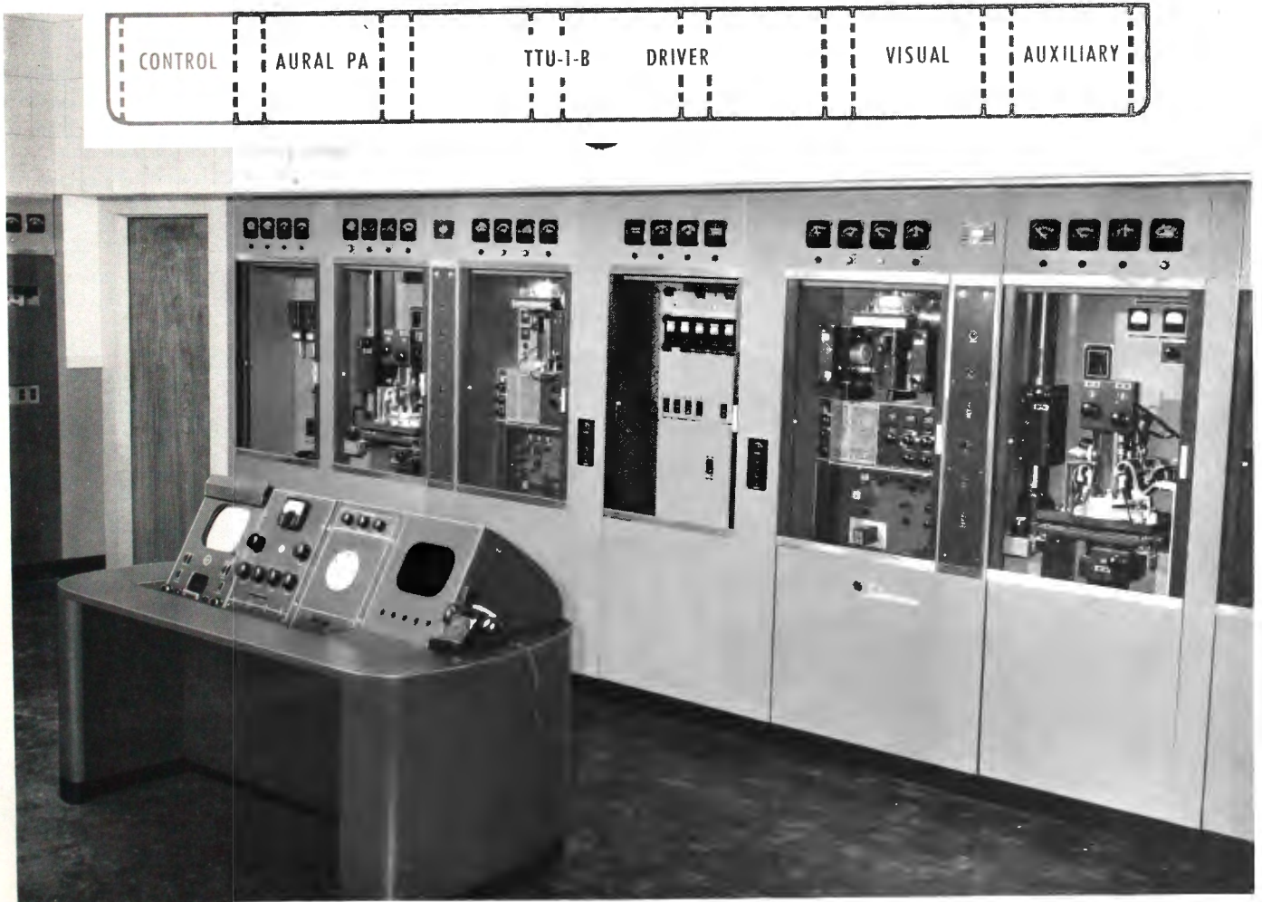
WBRE-TV's original TTU-12A Transmitter. The unit required slight modification in the aural P.A. so that this cabinet now provides the peak aural signal required for 25 kw operation. This transmitter serves as the driver chain for the amplifier pictured on the left hand page. Note that the TTU-1B is still an integral part of the new equipment.
