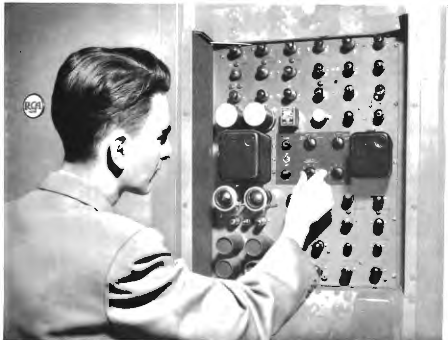
FIG. 9. View of the advanced design Sync Generator which has reduced the rack space to one-third that occupied by former designs. Providing extra stability, small size and combining all sync functions in a single chassis, it is ideal for color TV applications. It includes a built-in Genlock, dot generator, grating generator and regulated power supply.
